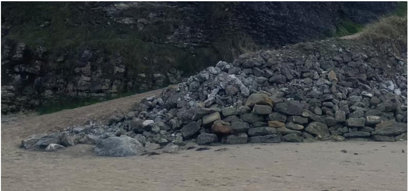
Figure 2.5 Rock armour at the lower portion of the existing access route
