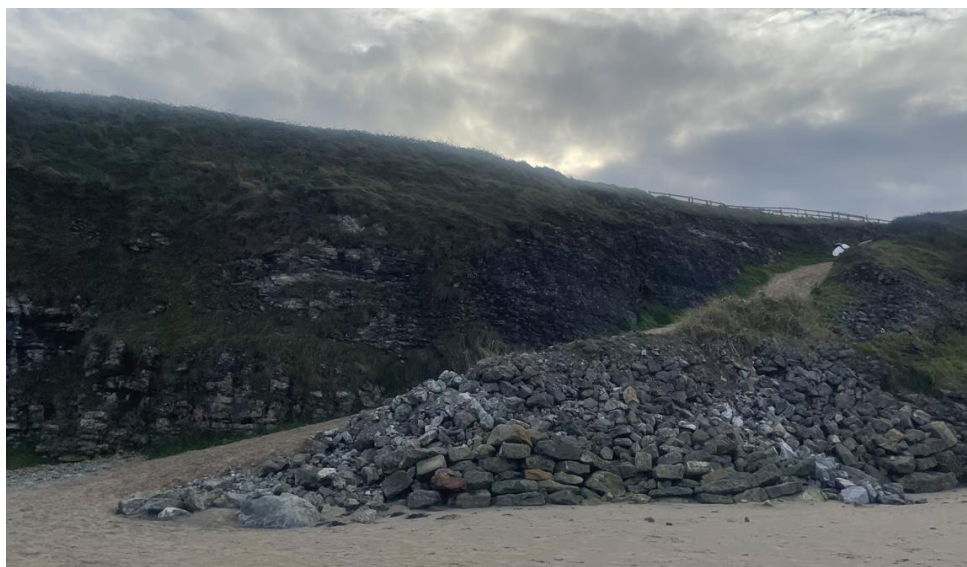
Figure 2.2 Existing Unauthorised Access to Tullan Strand
